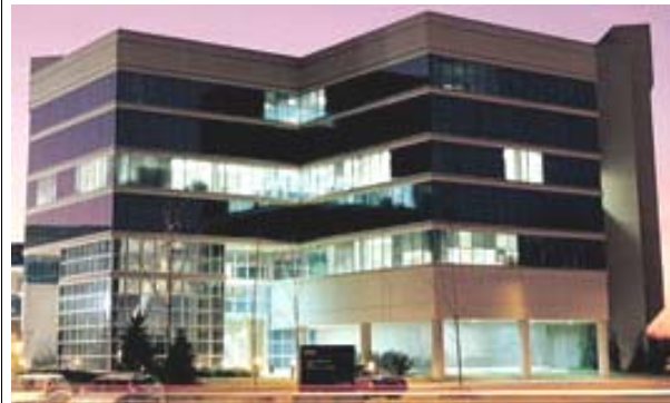
UAH Optics Building and Center for Applied Optics
